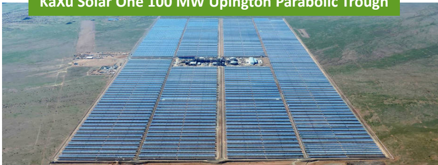
KaXu Solar One 100 MW Upington Parabolic Trough
