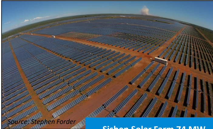
Sishen Solar Farm 74 MW
