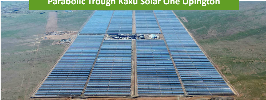
Parabolic Trough Kaxu Solar One Uppington
